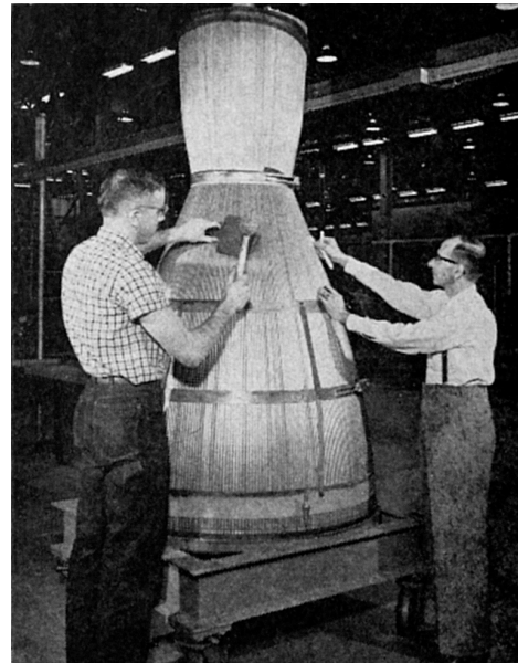
Figure 2 Brazed tube combustion chamber undergoing assembly (Image: Google Images)
