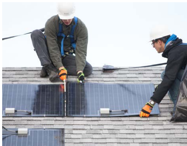
Figure 1: Installation of lightweight adhesively-mounted modules on a steep-slope shingled roof.
