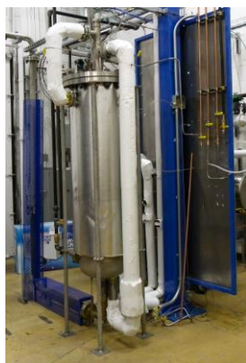
Figure 2: 10 BPD Plasma Natural Gas Reformer
