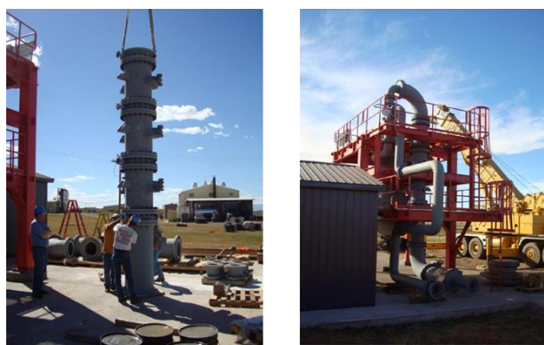
Figure 3: Reformer for biomass gasifier residuals
