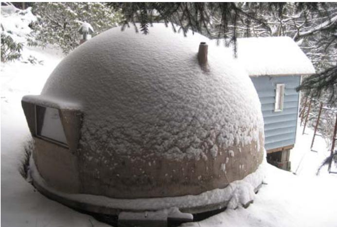
Figure 2. First prototype, insulated, with insulated floor. Total weight 1,050 kg. Juneau, Alaska
