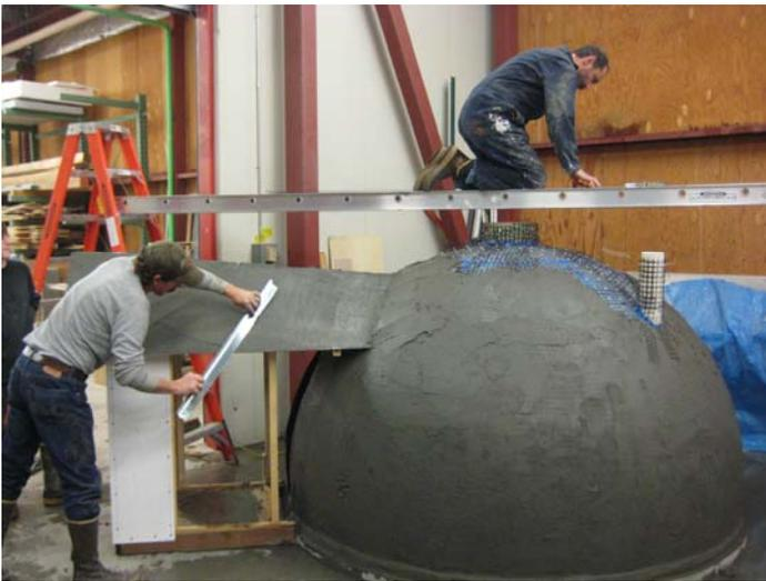
Figure 7. Applying mortar ~ 1 cm thick
