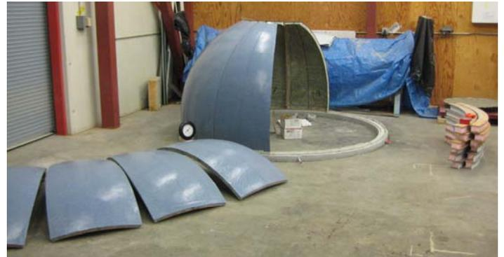
Figure 4. Assembling the dome form to the foundation ring. A shim 3/8" thick is installed between pairs of form "orange peel" segments
