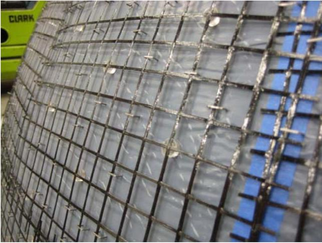
Figure 6. C-Grid attached to dome form segments with stainless steel staples. Note clear plastic “chairs” to space C-grid ~ 1 / 2 cm from Teflon surface.
