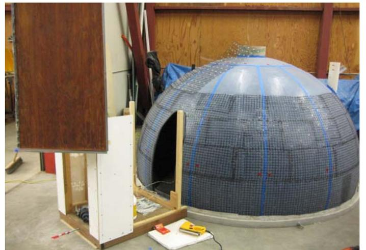
Figure 5. Stapling "tiled" C-Grid to dome form
