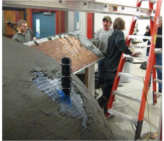
Figure 8. Applying mortar ~ 1 cm thick
