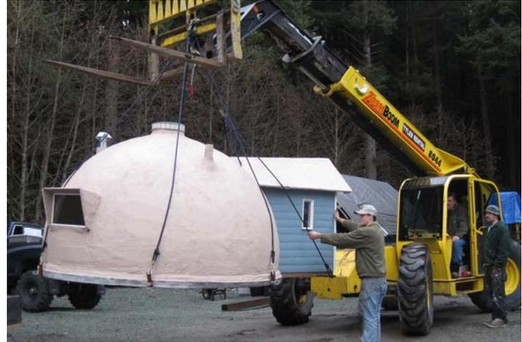
Figure 3. First prototype, insulated, with floor. Total weight 1,050 kg.
