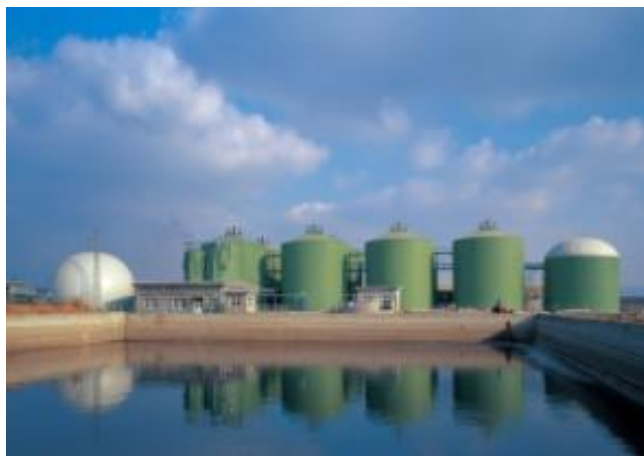
Fig. 4a. A centralized communal chicken waste treatment facility producing electricity for local network.
