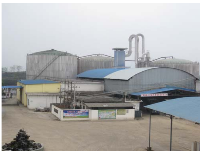
Fig 5. The alcohol producing facility using UASB processes to produce methane-rich biogas.
