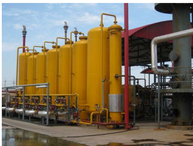
Fig 3. Biogas purification facility producing methane with 97% purity.
