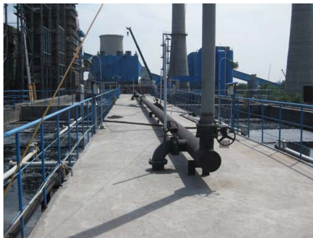
Fig. 1. The top of the UASB reactor treating starch wastewater.
