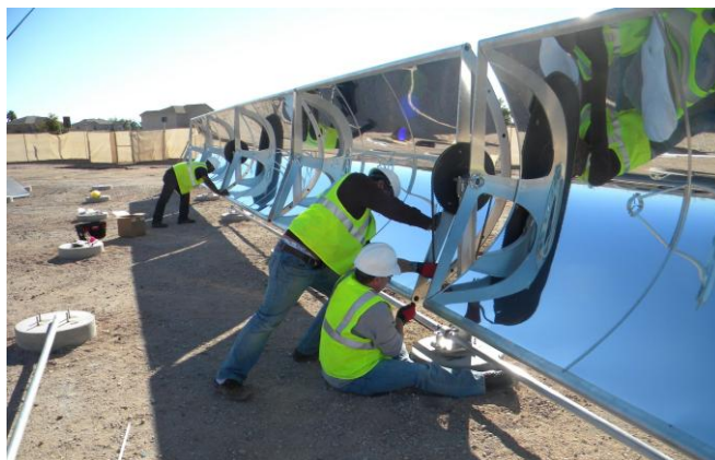
Figure 1: Local labor installing MicroCSP collectors at Davis-Monthan Air Force Base in Arizona.
