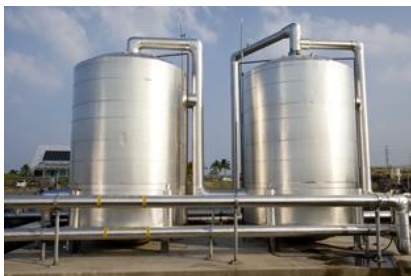
Figure 4. Thermal storage at Holaniku, Kona, HI
