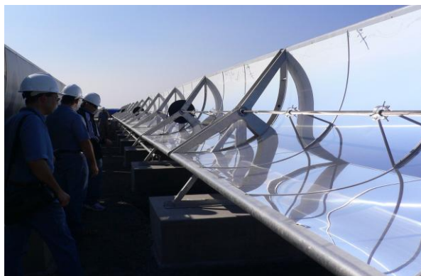
Figure 1: Sopogy's MicroCSP collectors at Holaniku
