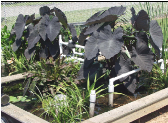
Figure 2. Small ReCip® “water garden” designed to treat up to 300 gal. per day (appropriate for a single
