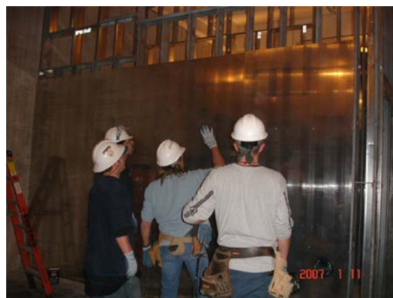
Figure 9: Six sided EM room shield installation at a University Microscopy Center. [4]
