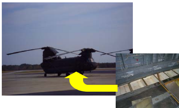
Figure 2: CH-47 Chinook Corrosion Under Floor Boards
