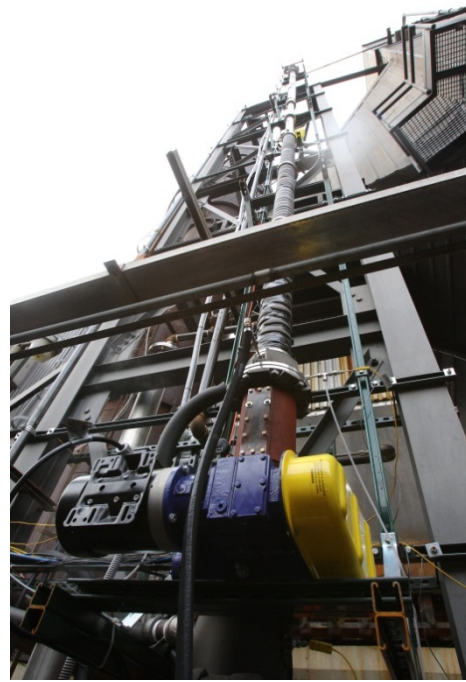
Figure 4: Field pilot column at the University of Toledo.
