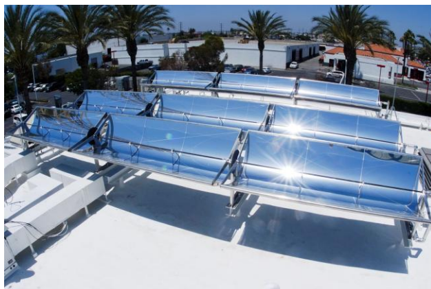
Figure 1: MicroCSP tracking sun in southern California to partially fuel a solar air conditioning system
