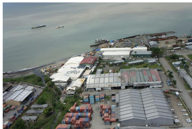
Figure 7: Solar hot water and process heat installation, Frabelle tuna factory, Oct. 2011, Papua New Guinea
