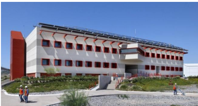
Figure 3: MicroCSP collectors on roof of Holcim-Apasco Cement Building in Hermosillo, Mexico
