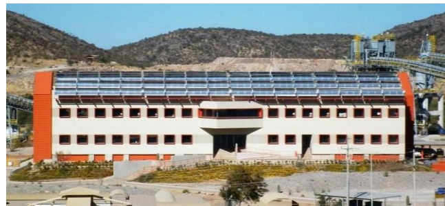
Figure 5. Holcim Apasco’s roof top MicroCSP installation
