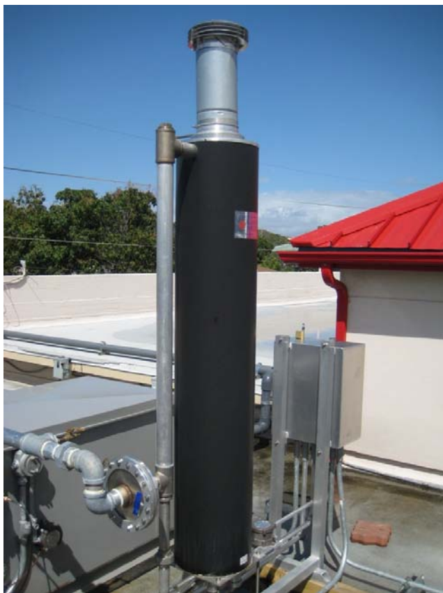
Figure 2: Electric Catalytic Oxidizer Installed On The Roof
