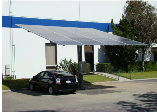
Figure 3: Center post carport
