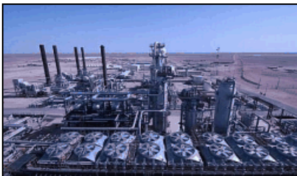
Figure 6 : CO 2 project in Algeria.
