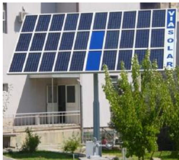
Figure 7: General view of 3.1 kWp tracking PV water pumping demonstration system.
