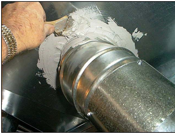
Fig. 4 Duct work being properly sealed with mastic
