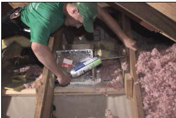
Fig. 2 Air Sealing an Insulated Box over a Recessed Can Light
