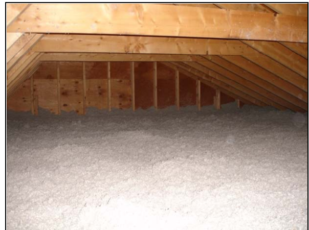
Fig. 3 Super Insulating the Attic
